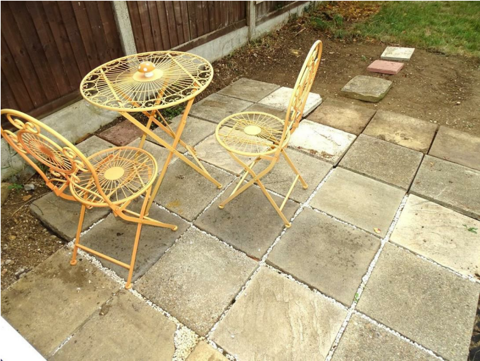
PAVED PATIO AREA
