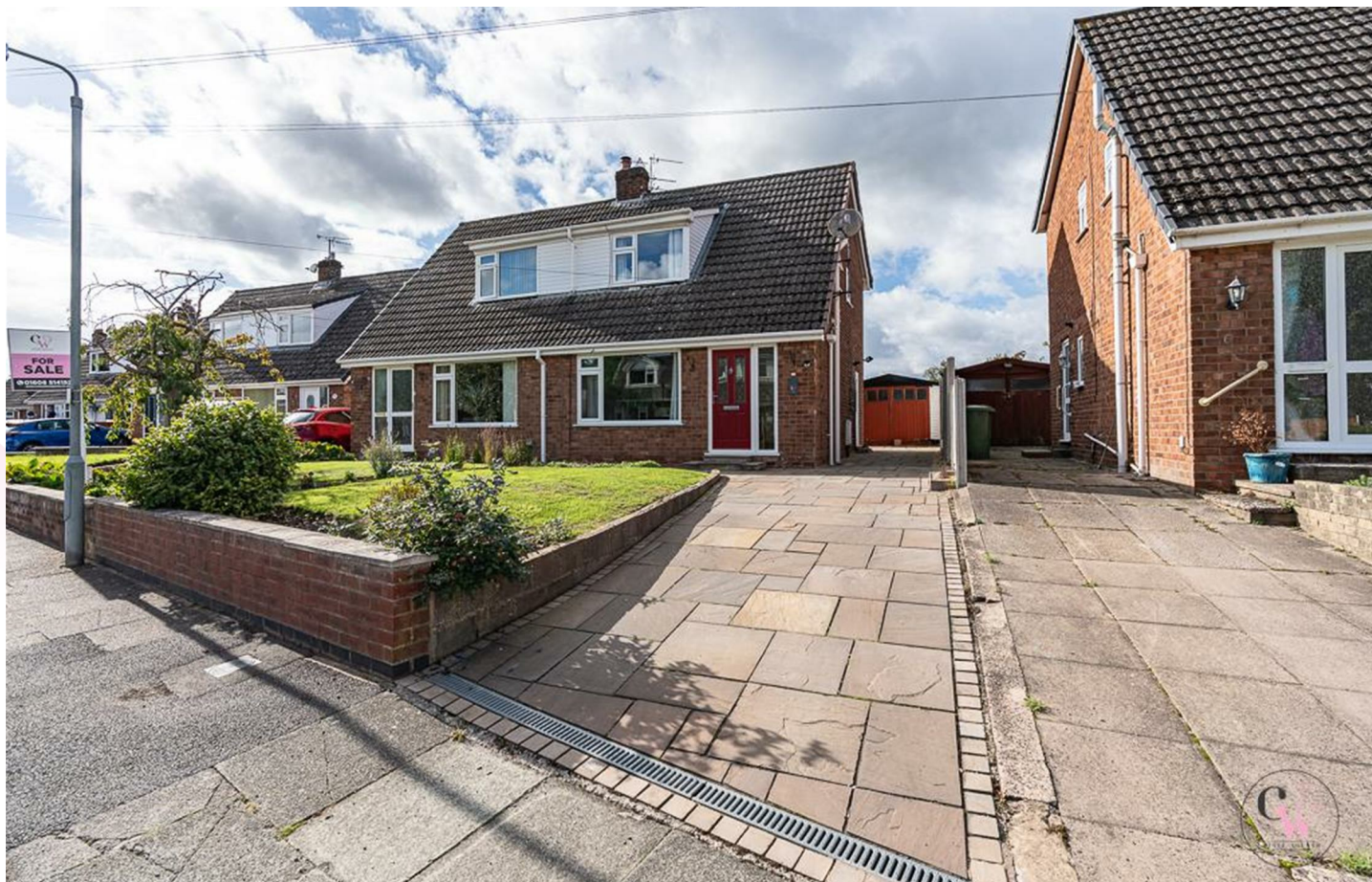
Sandyhill Road, Winsford CW7 1JL
