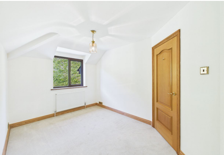
Door into hallway.
