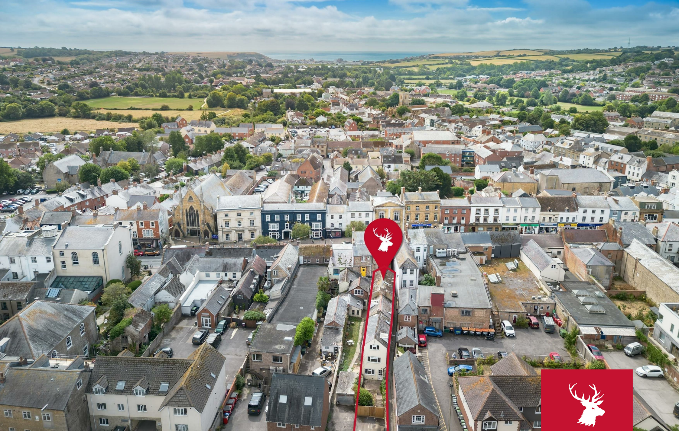
9 Rax Lane and Adjoining Building
