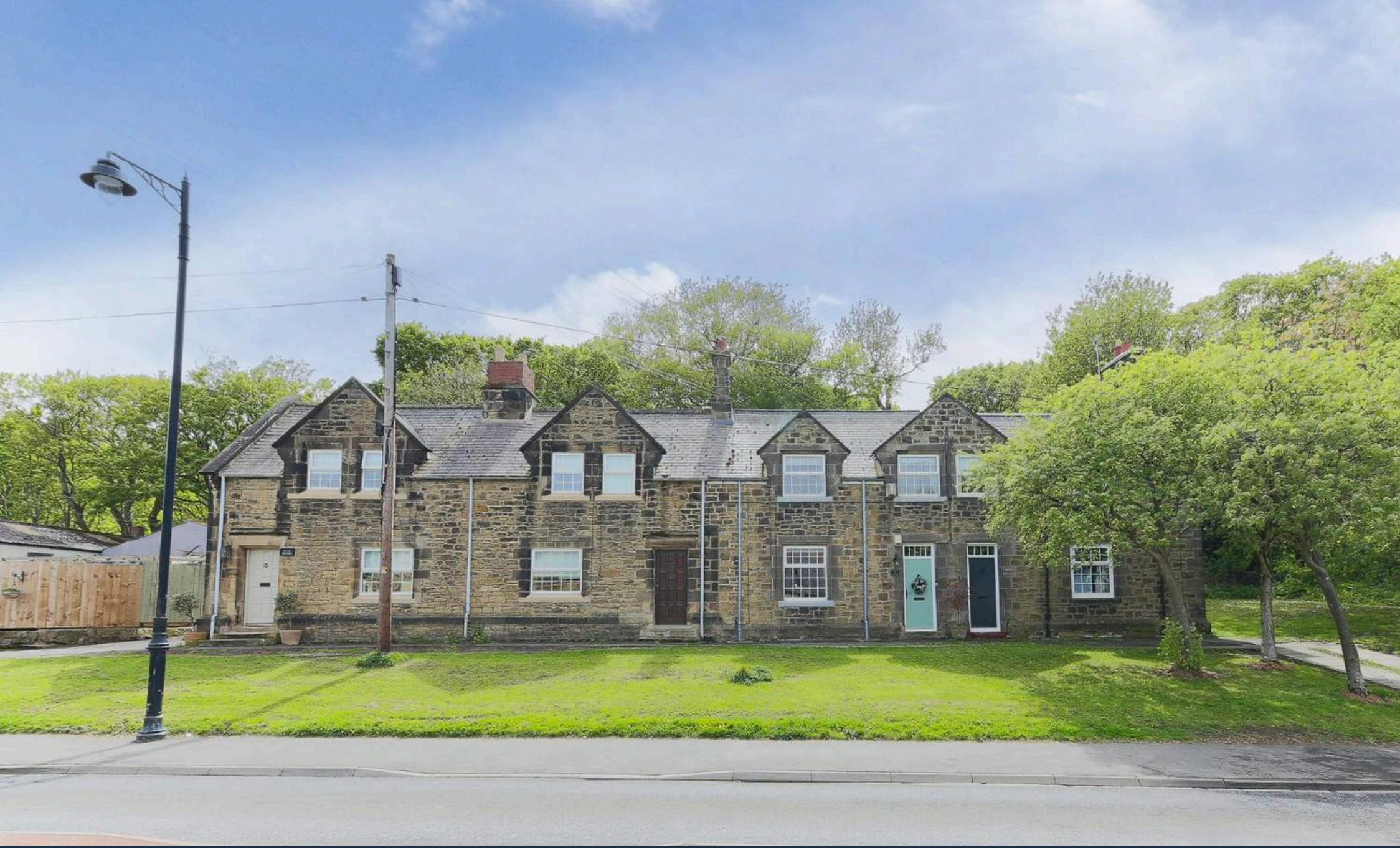
2 West Cottages, Backworth Newcastle Upon Tyne
