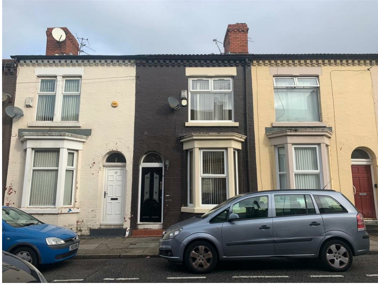
With forecourt to front of property
