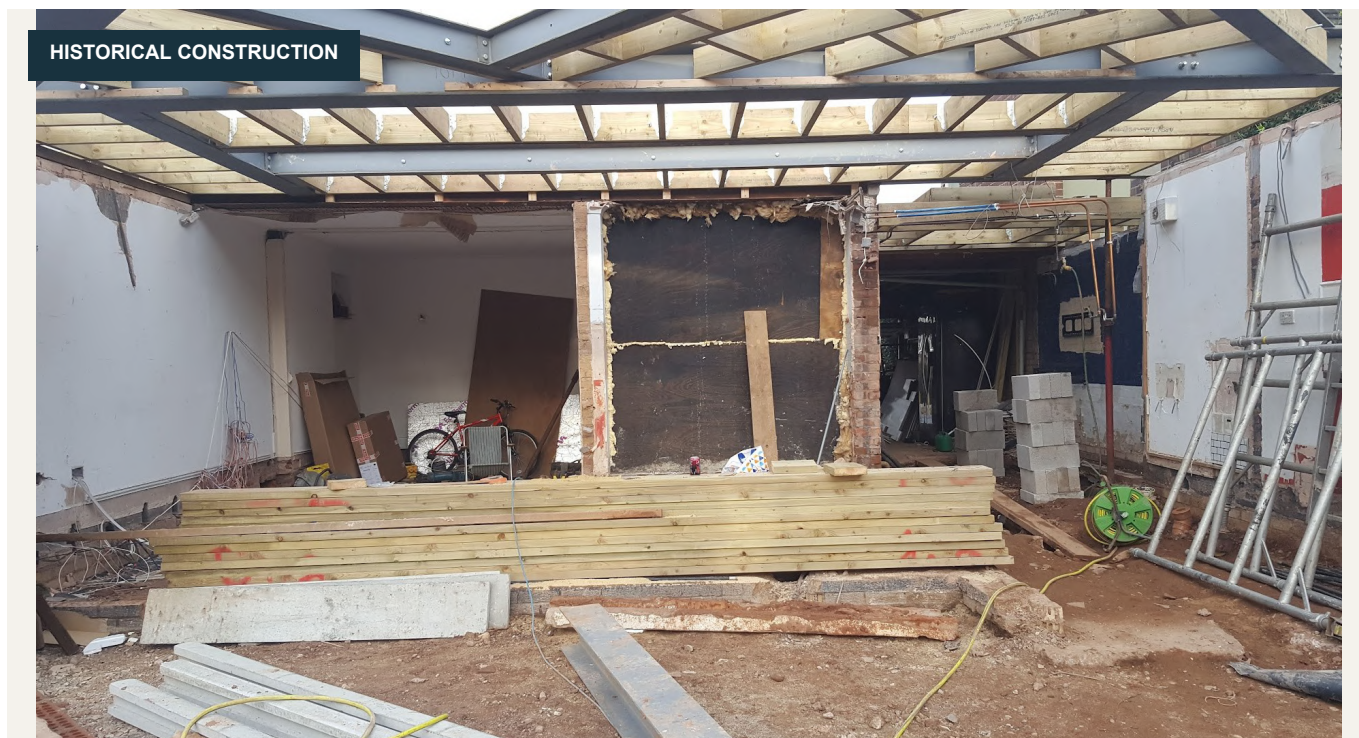
5 February 2020: timber joists and framed roof openings over the rear extension.
