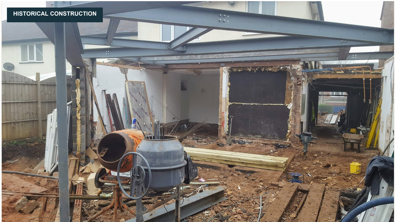
23 January 2020: the installed steel frame, viewed towards the house.
