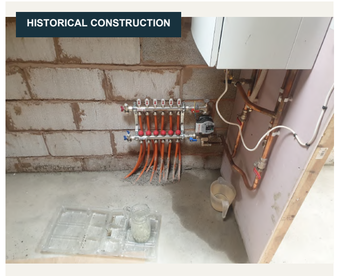
20 June 2021: heating manifold and boiler installation.
