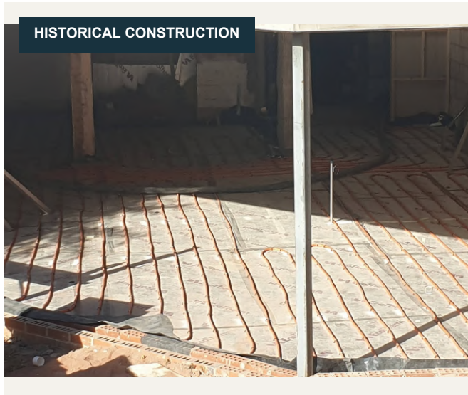
15 June 2021: installed underfloor-heating pipework before covering. Vendor-supplied image.
