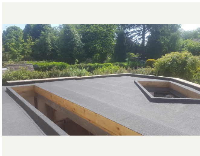
27 May 2020: weather-protected roof deck and formed openings.
