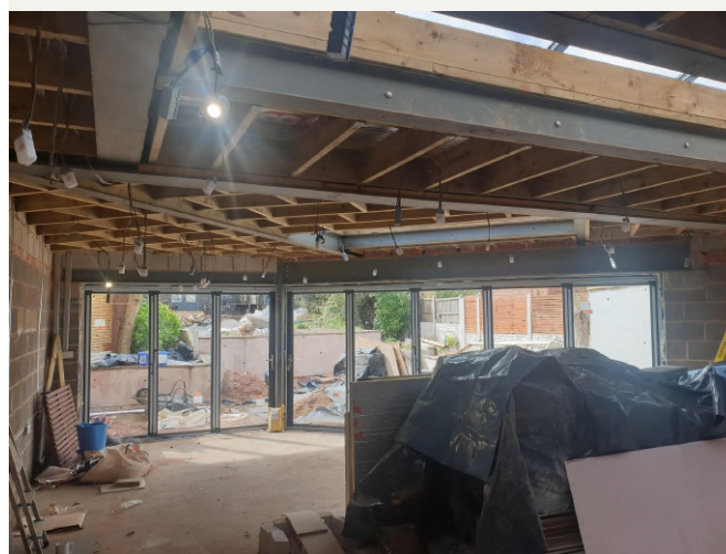
6 April 2022: internal structure and rear glazing during fit-out.
