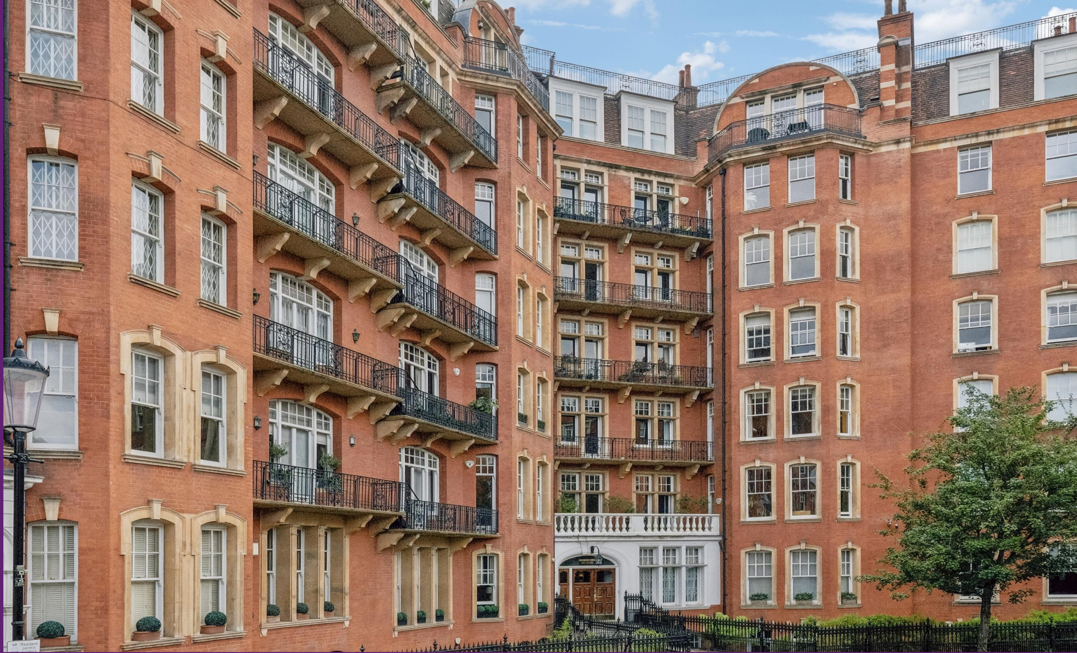
Oakwood Court Kensington, W14
