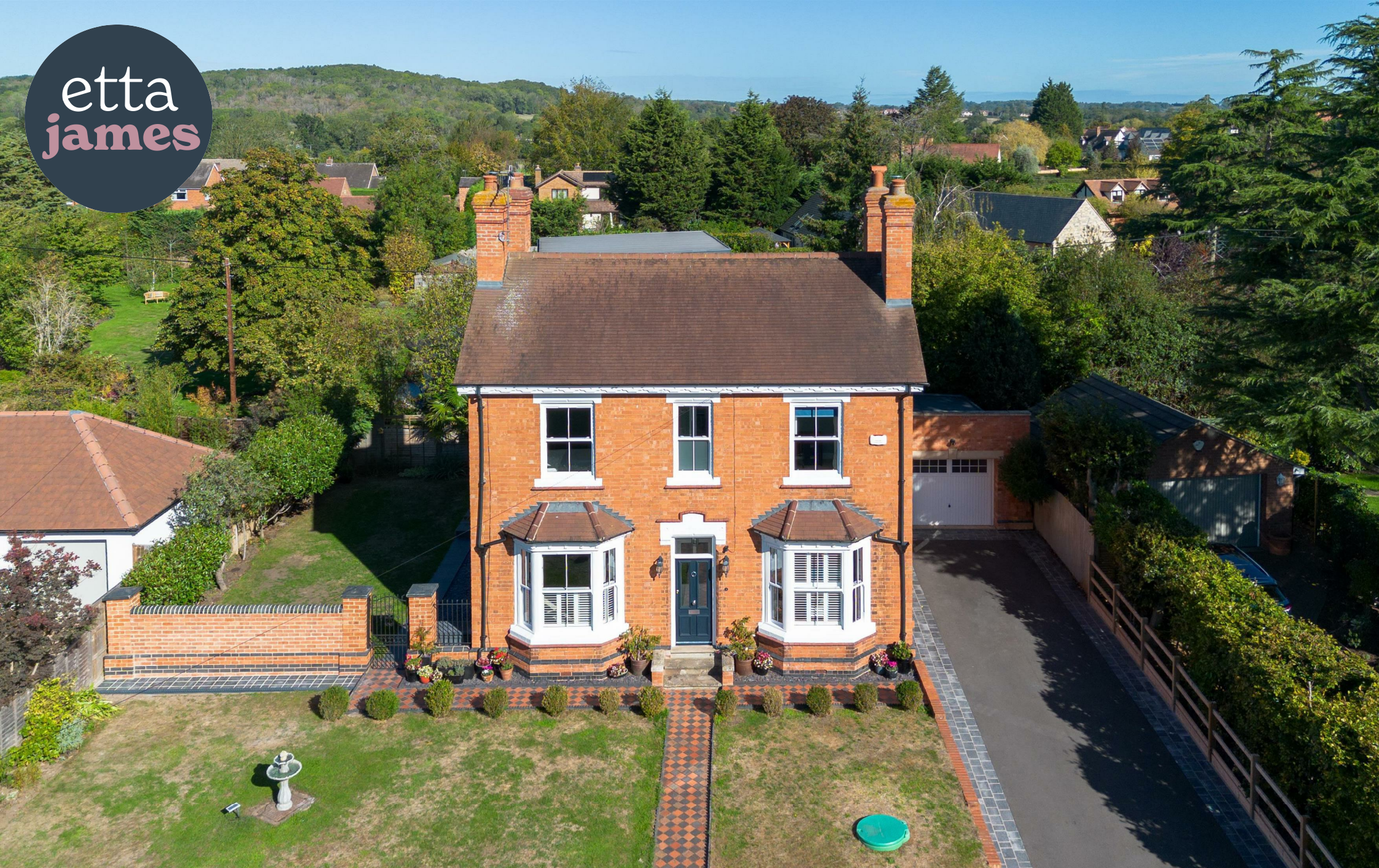
CHURCH STREET, WELFORD ON AVON, CV37 8EJ
