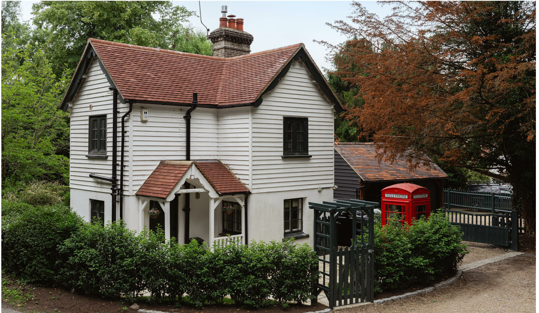
Church Road, Horley
