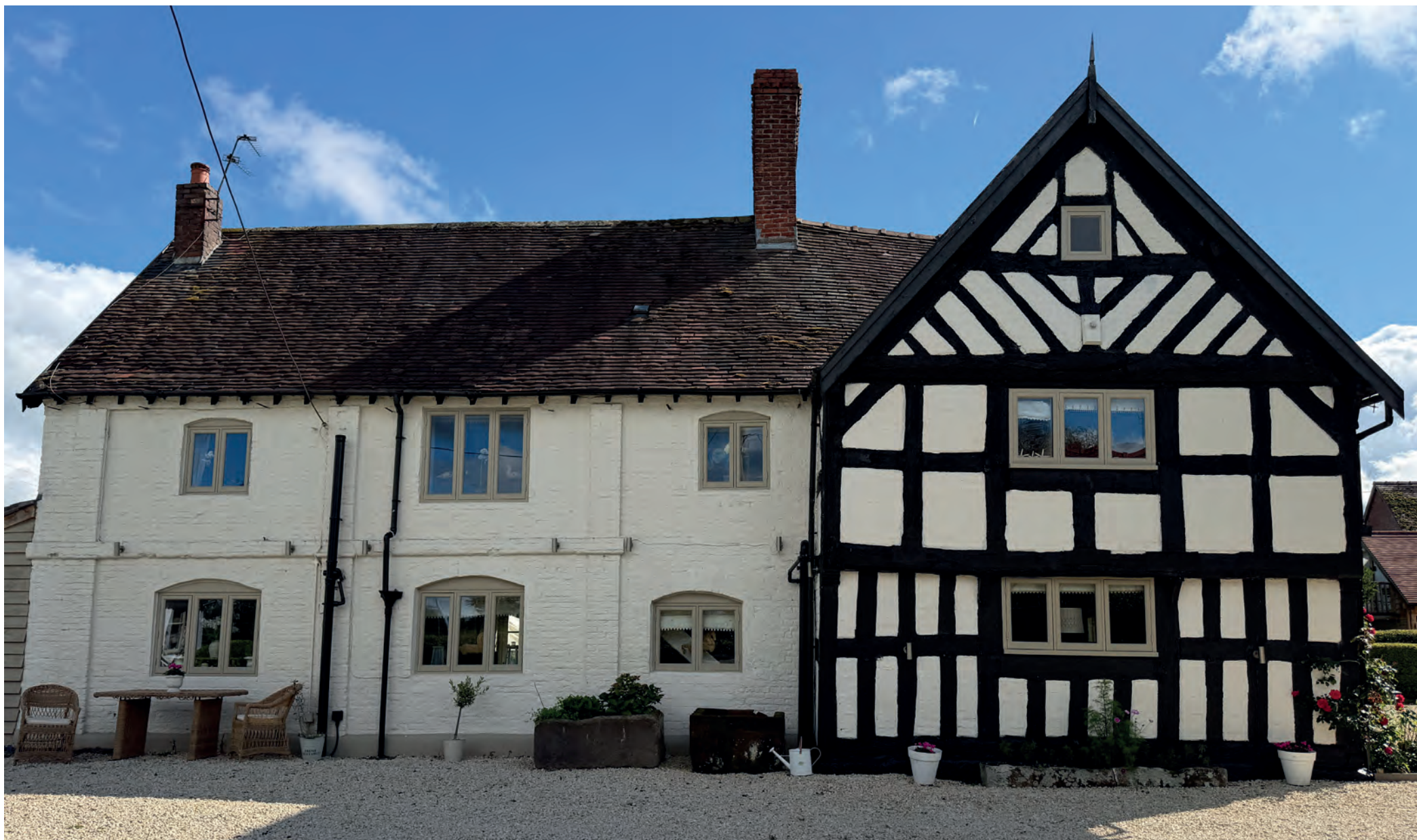
Spensford House Loppington | Shrewsbury | Shropshire | SY4 5NG
