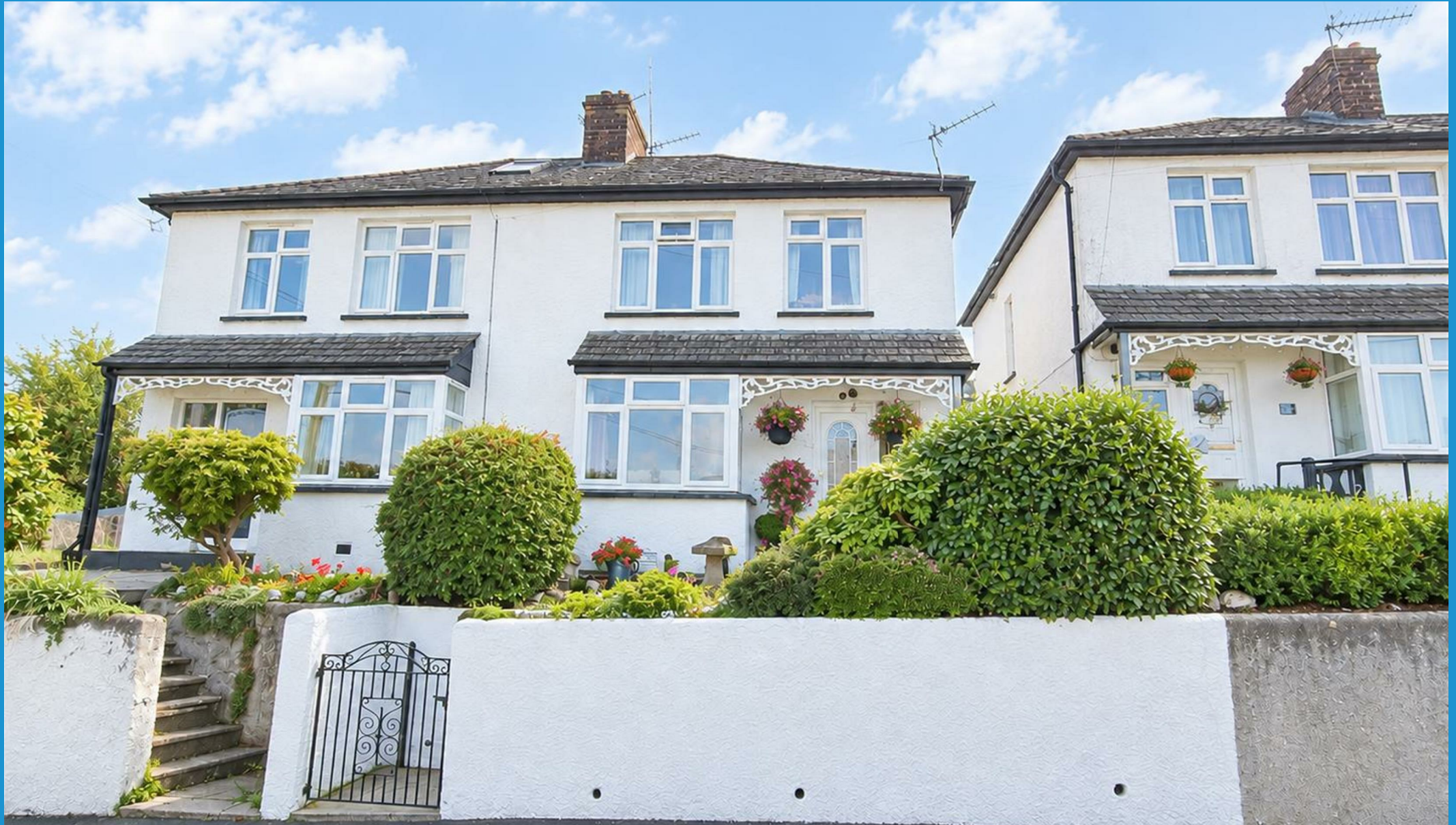
Priory Park Road Launceston | Cornwall
