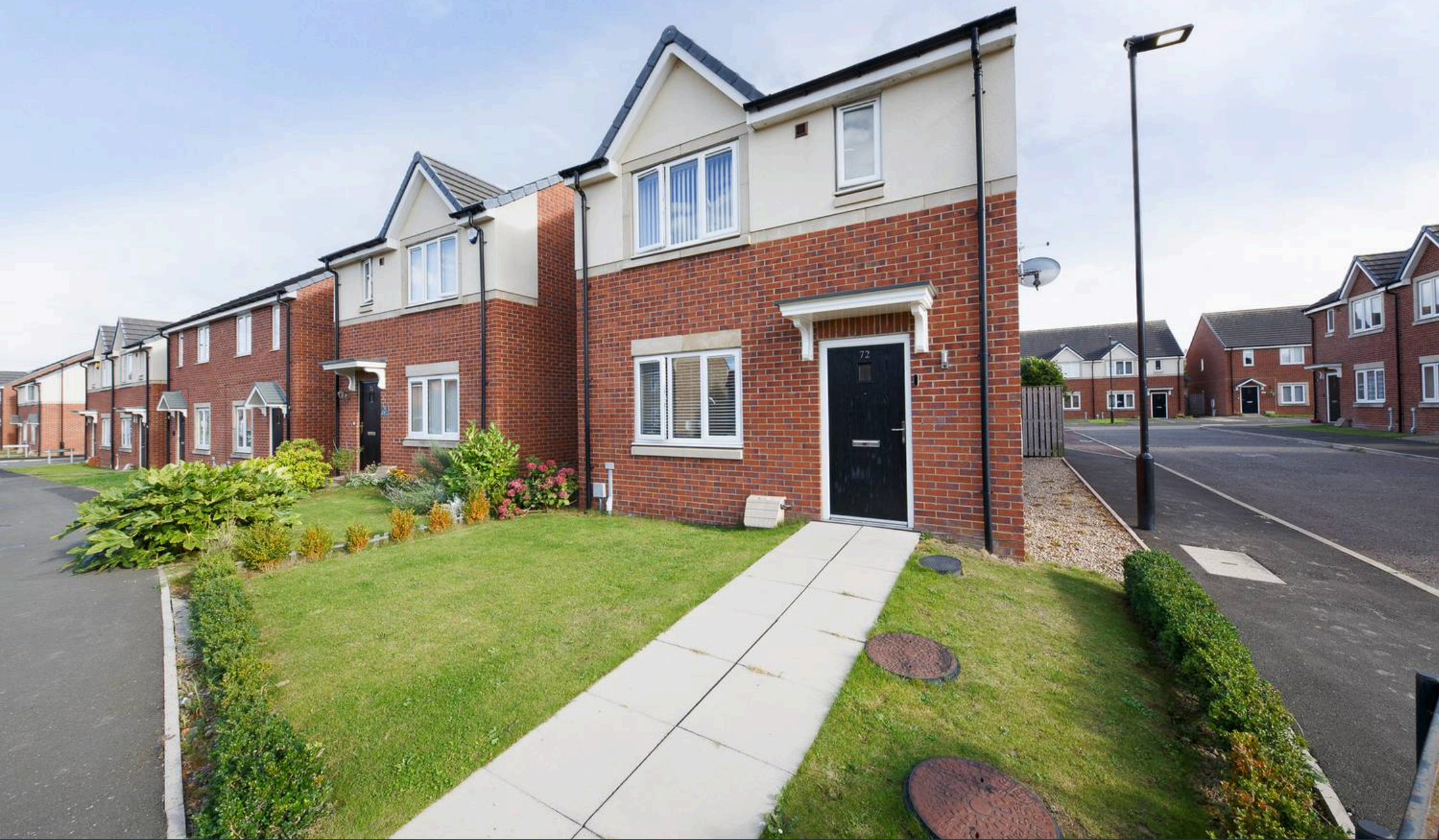
72 Hotspur North, Backworth Newcastle Upon Tyne
