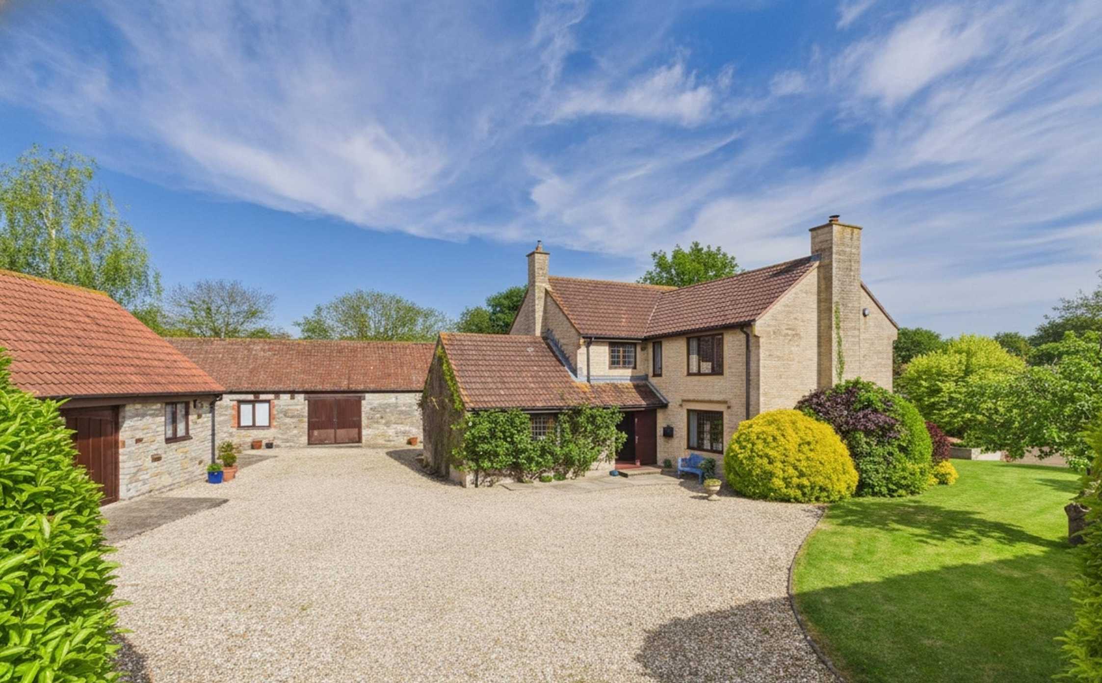
Old Church Farm House School Street, Drayton, TA10 0LH
