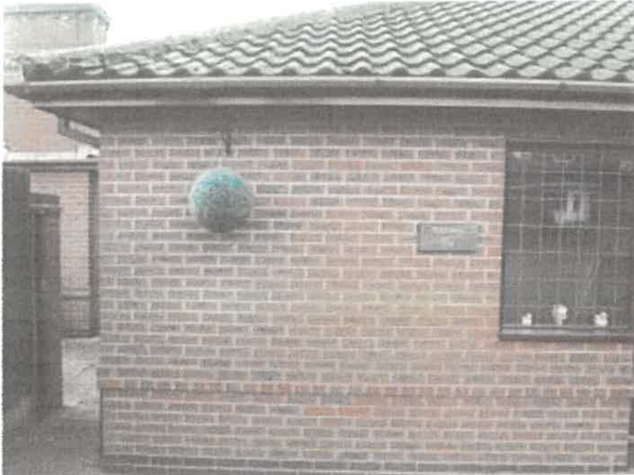
Photograph 1 – Front LHS wall elevation
