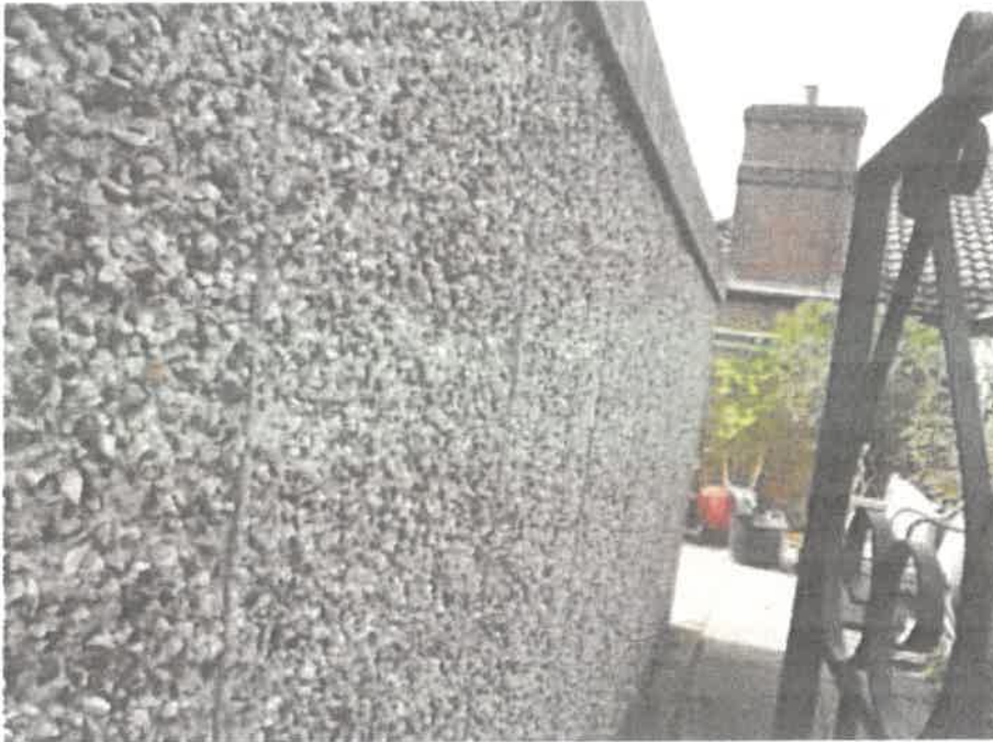
Photograph 10 – RHS gable wall to garage
