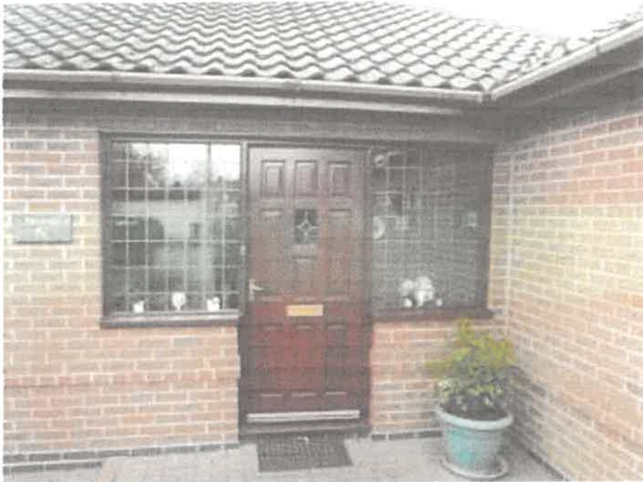
Photograph 2 – Front RHS wall elevation
