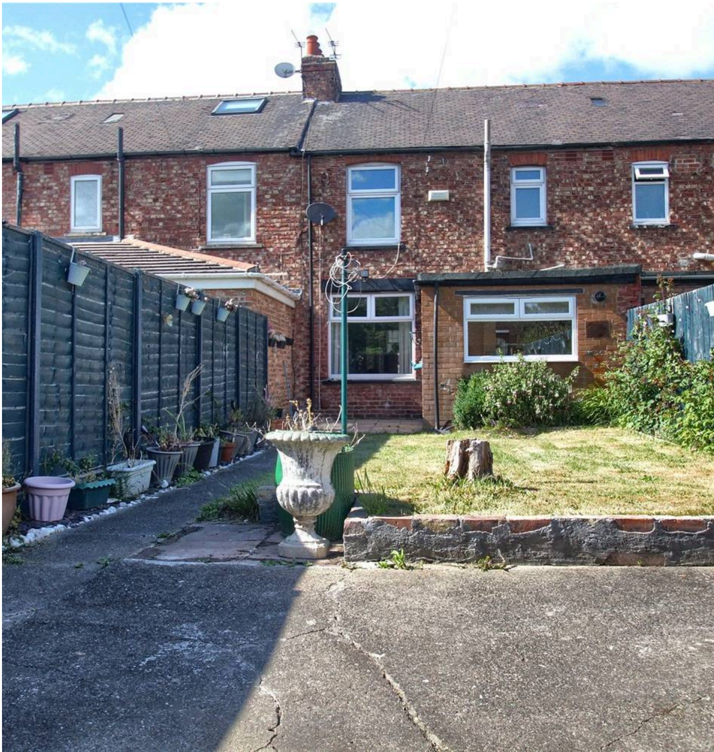
16 Oxford Road Middlesbrough
