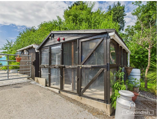
2 cat rooms to the right hand side of the main building.
