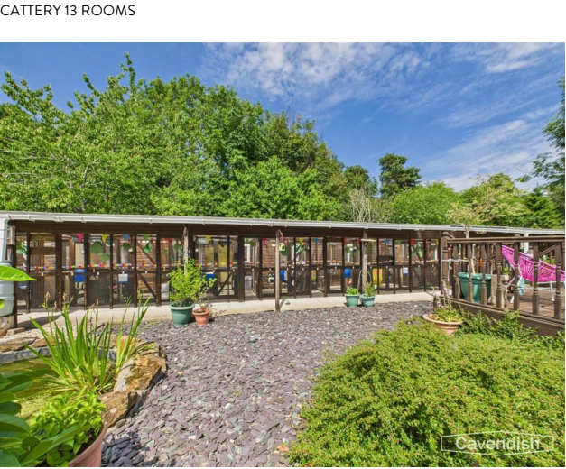
13 additional cat rooms located to the rear of the main building. THE COTTAGE
